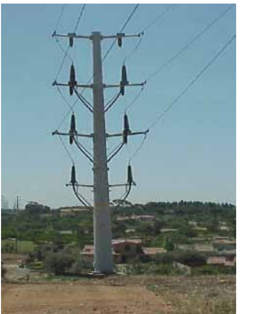
Steel termination pole
