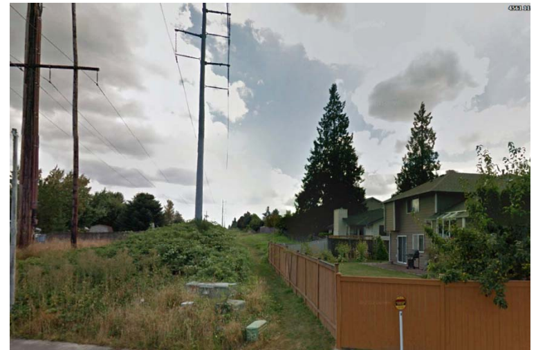
230 kV transmission line in Everett, WA
