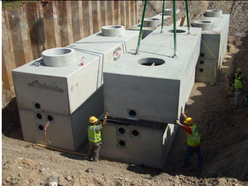
Figure 2-9 Splicing Vault Installation
