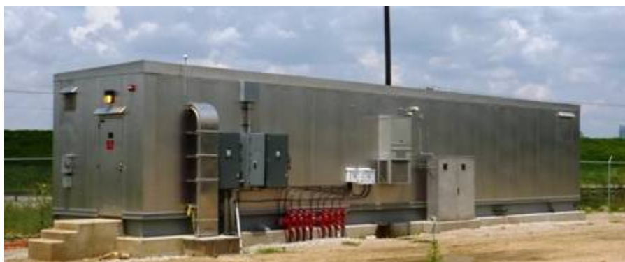
Figure 2-15 Typical Pressurization Plant
