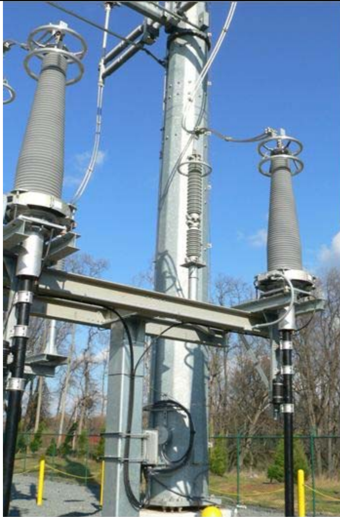
Figure 2-3 Typical 230 kV XLPE Terminations
