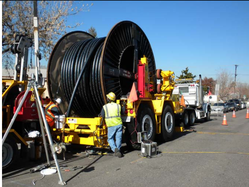
Figure 2-10 Typical Cable Pulling Set up
