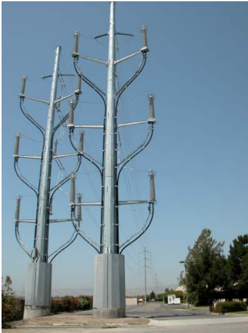
Figure 3-10 Typical 230 kV Riser Structure
