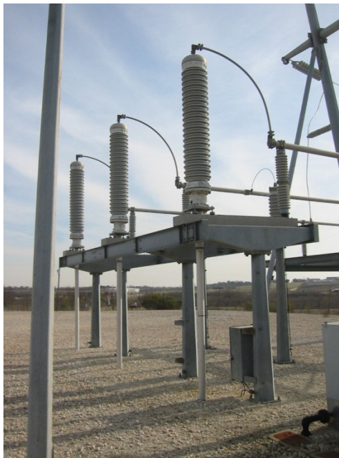
Figure 2-13 Typical HPFF Terminations in a Substation
