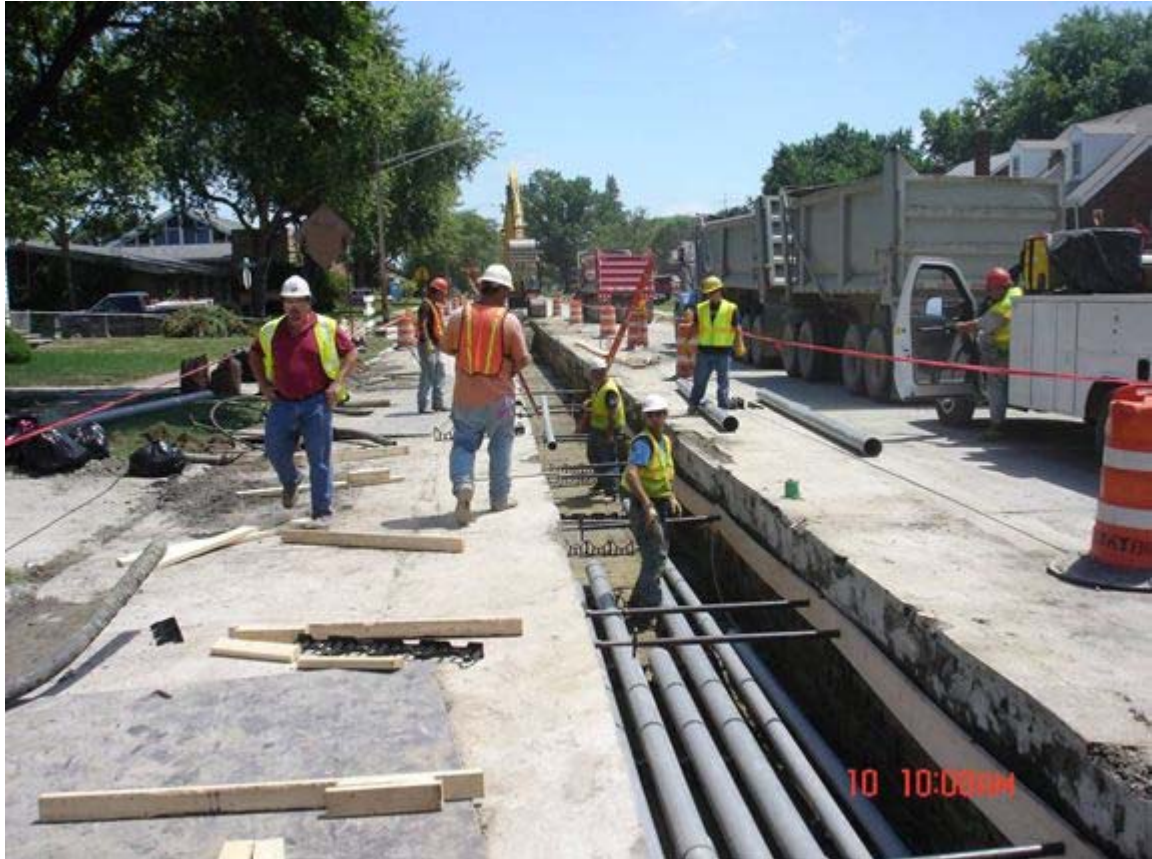
Figure 2-4 Typical trench excavation and duct bank installation (city street)
