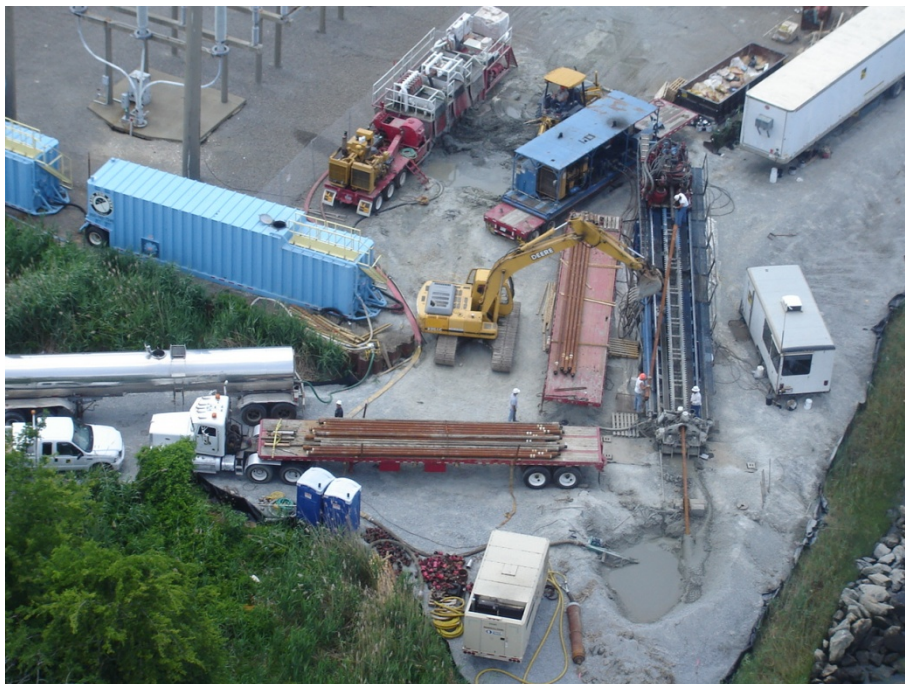
Figure 2-7 Typical HDD Setup
