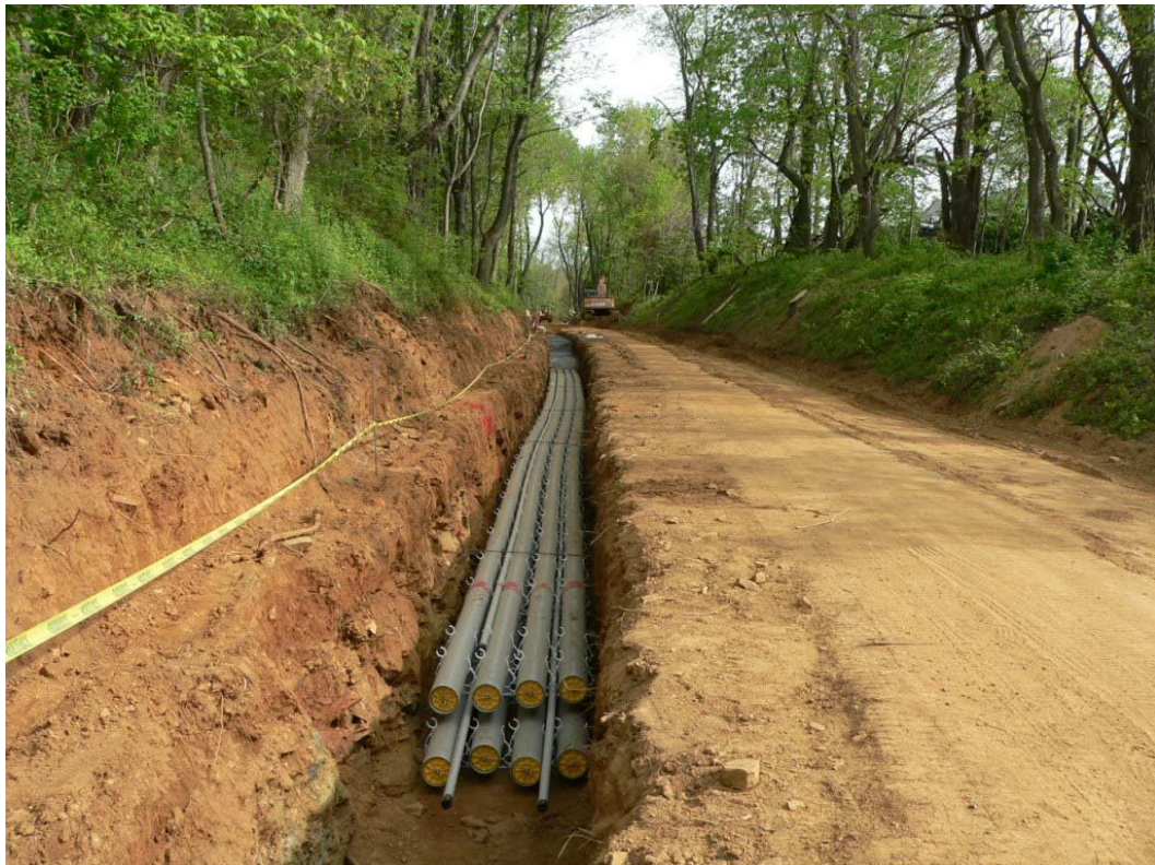
Figure 3-9 Example of duct bank construction in Railroad (retired) Corridor
