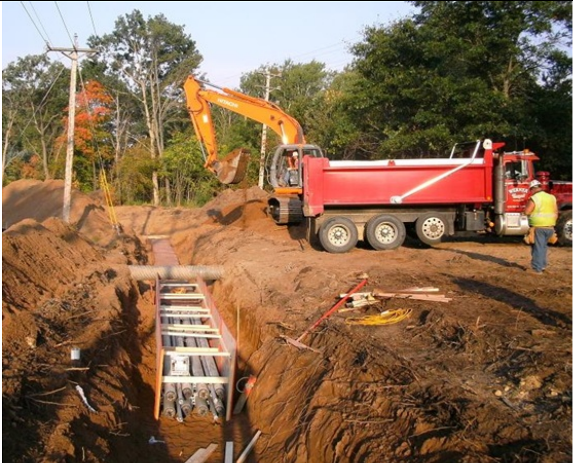
Figure 2-5 Typical trench excavation and duct bank installation (rural)
