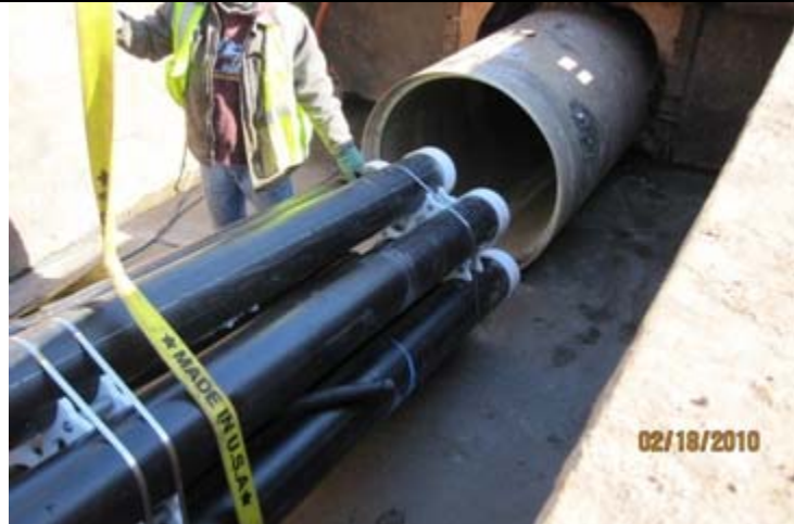
Figure 2-6 Typical Jack and Bore Conduit and Casing Arrangement
