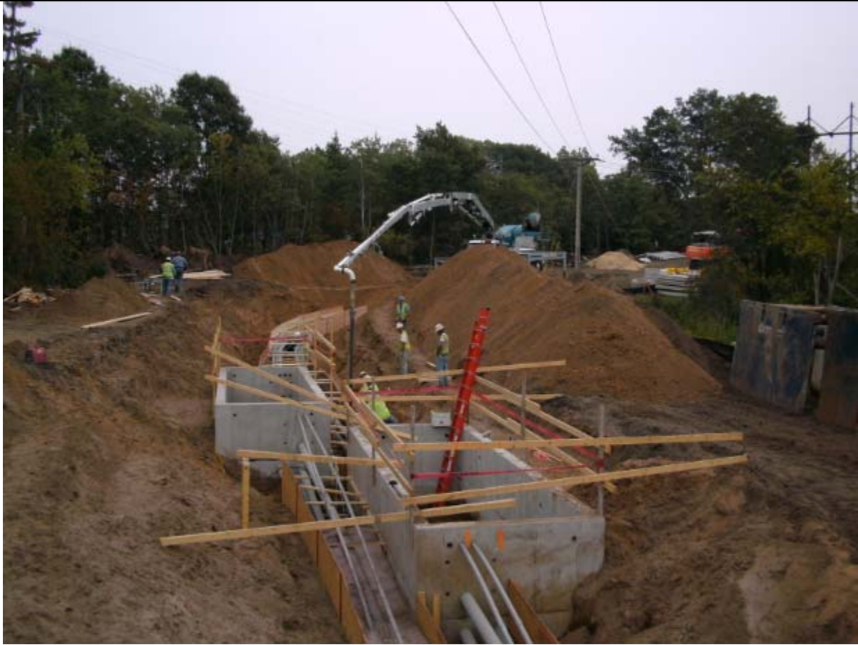
Figure 3-5 Duct Bank and Vault Placement in Rural ROW
