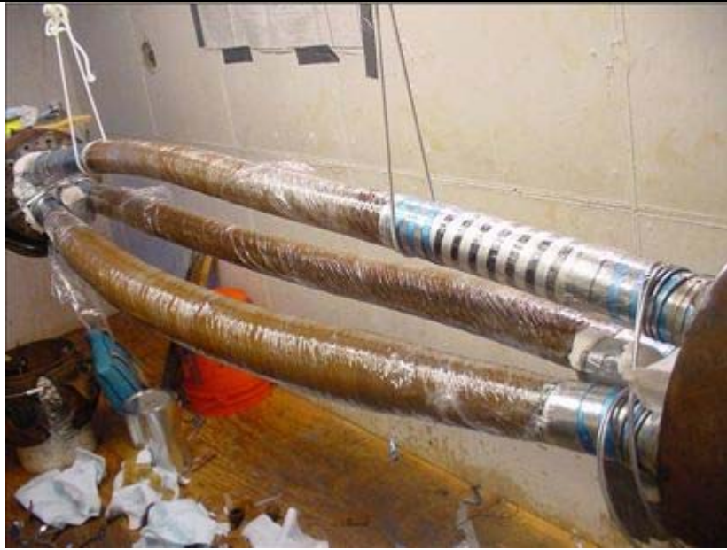
Figure 2-12 Typical HPFF Joint in a Vault
