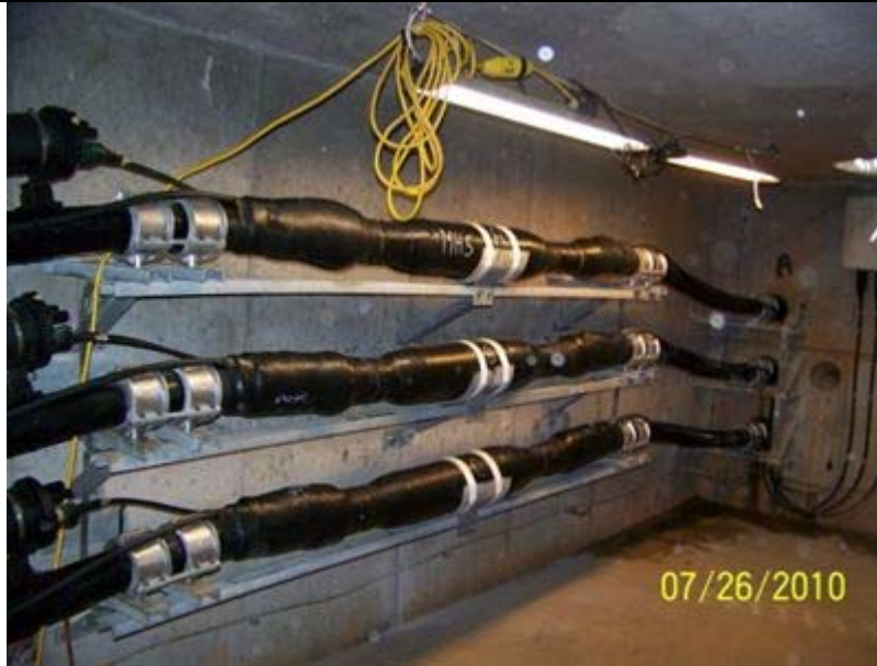
Figure 2-2 Typical 230 kV Pre-Molded XLPE Splices
