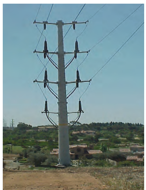
Steel termination pole
