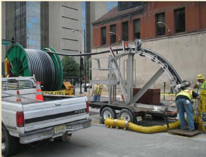
Cable being fed into the conduit system
