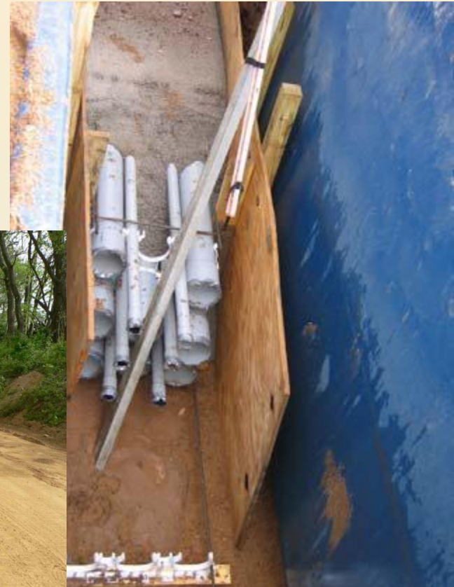
Conduit with thermal backfill installed
