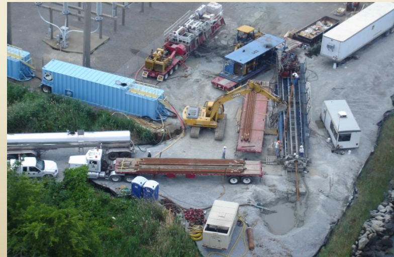
Horizontal Direction Drilling set up
