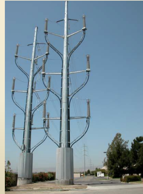
Double-circuit six-cable system
