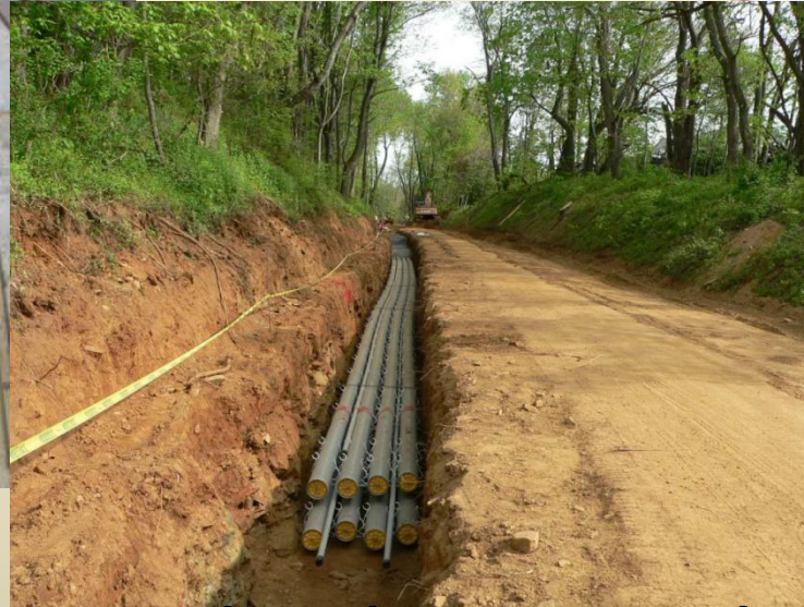
Conduit along a retired railroad corridor
