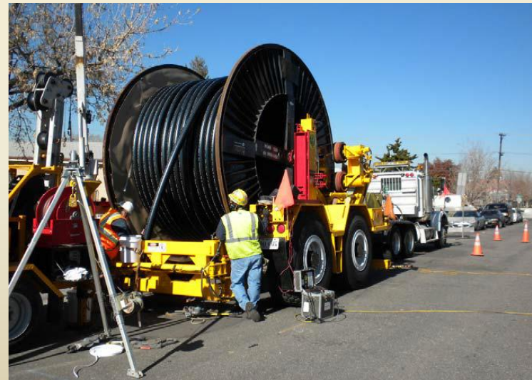
Cable being fed into the conduit system
