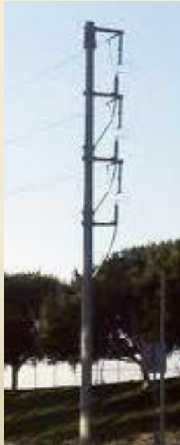
Single-circuit three-cable system
