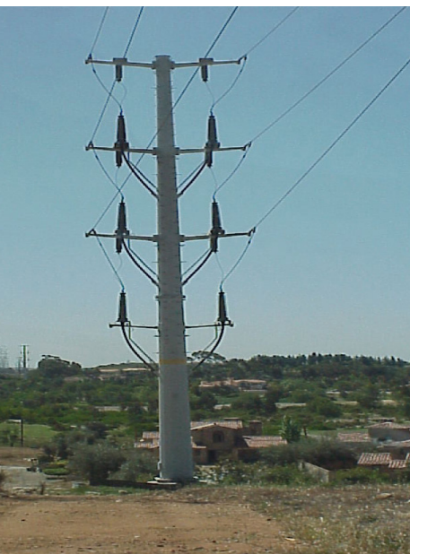
Steel termination pole
