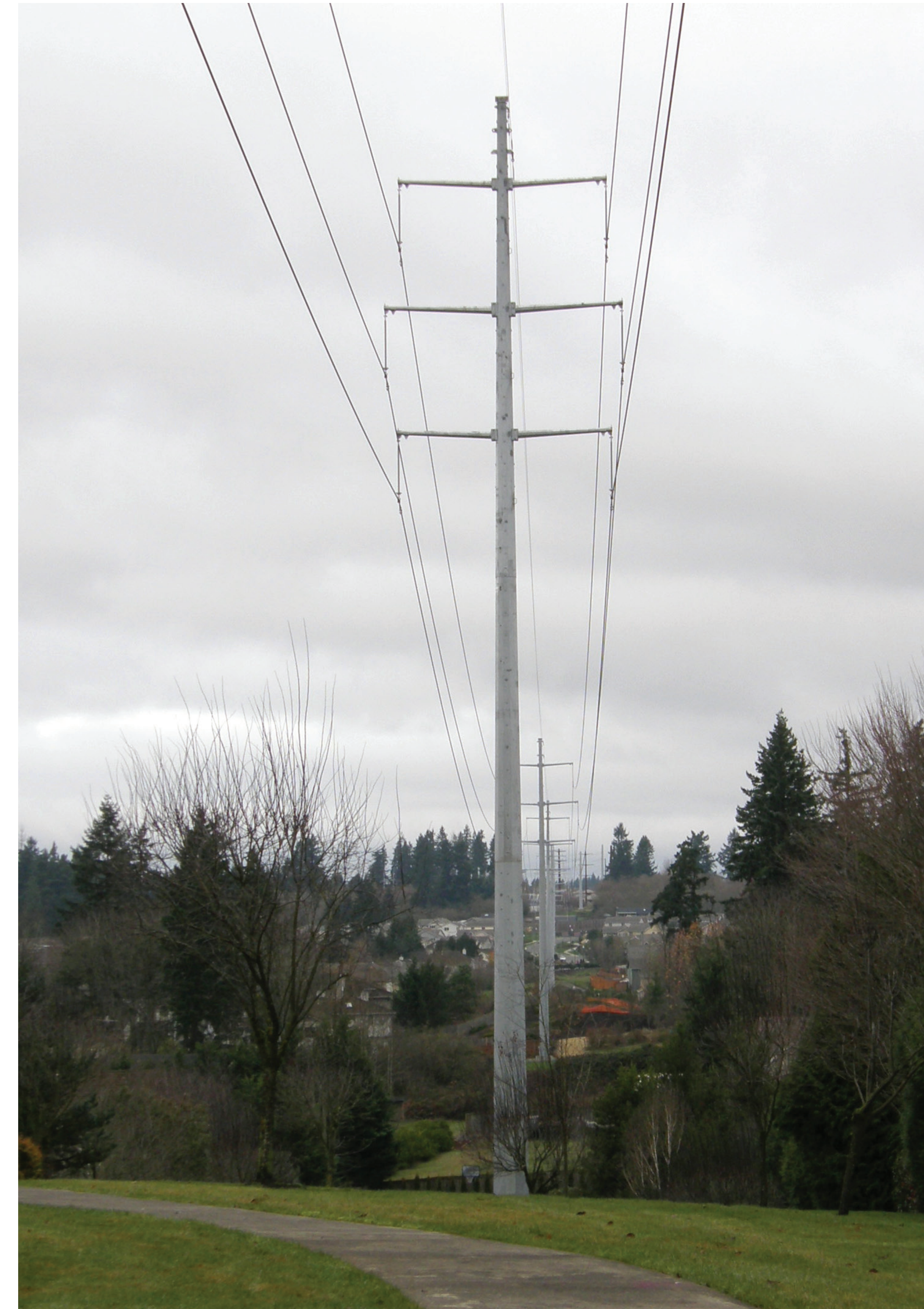
Double-circuit 230 kV steel pole
