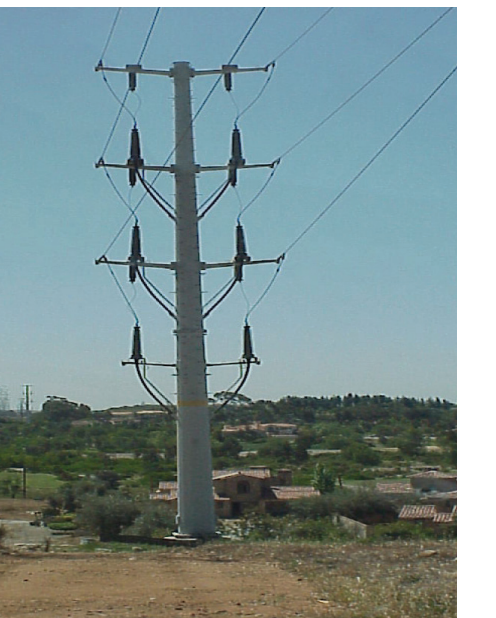
Steel termination pole
