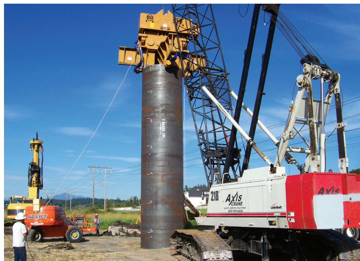
230 kV poles under construction
