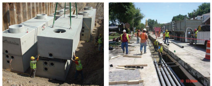
Construction of concrete duct bank for underground lines.
