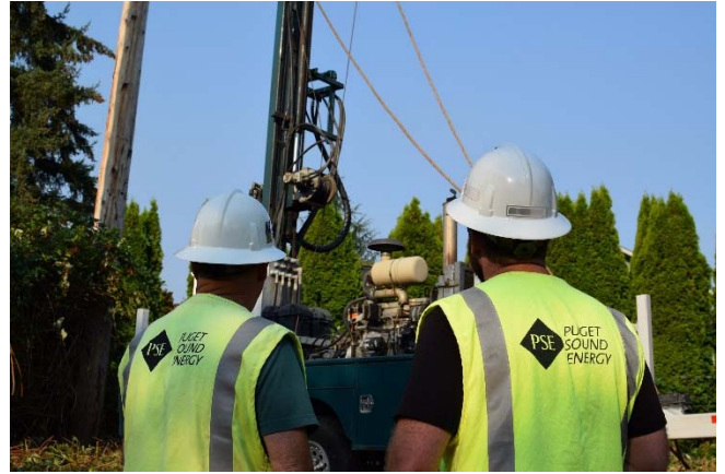
Geotechnical field crews completing a soil boring.
