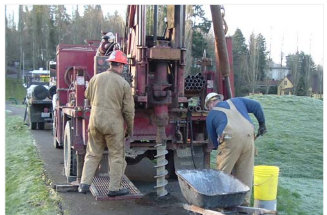
An example of a truck-mounted drill rig.
