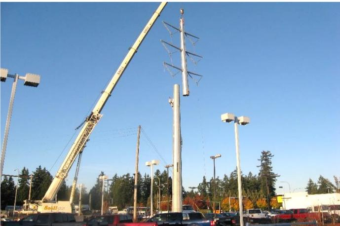
Typically, each new pole will be installed directly into the ground or placed on a concrete foundation, such as a drilled pier foundation or a self-supporting foundation. This will be determined by the structural loading, soil strength, and accessibility of each pole site. Installing drilled pier foundations will involve placing a reinforced-steel cage into the excavated hole and covering the cage with concrete.
