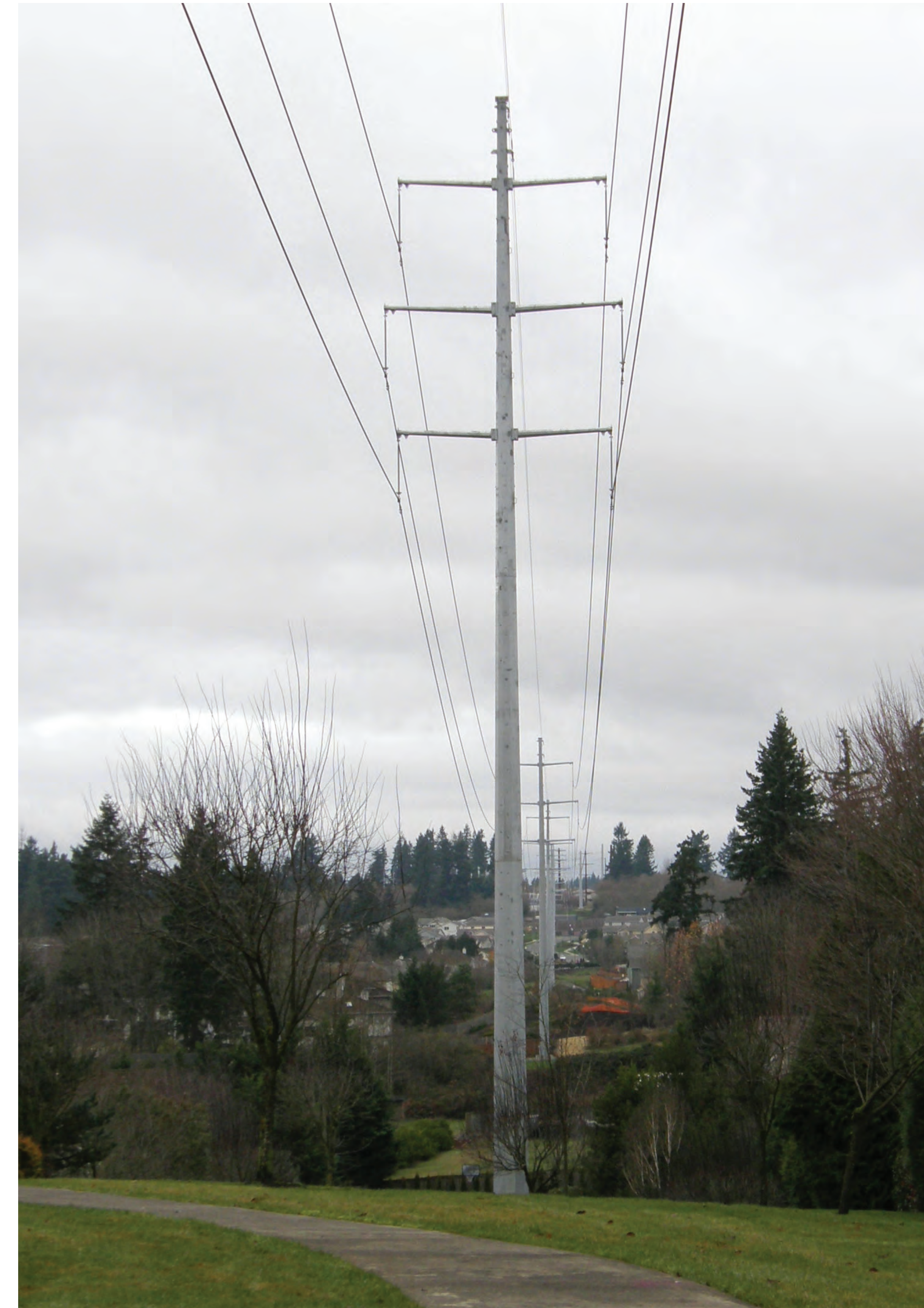
Double-circuit 230 kV steel pole
