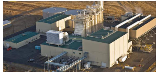
PSE's Goldendale generating station, a natural gas power plant in Klickitat County.
