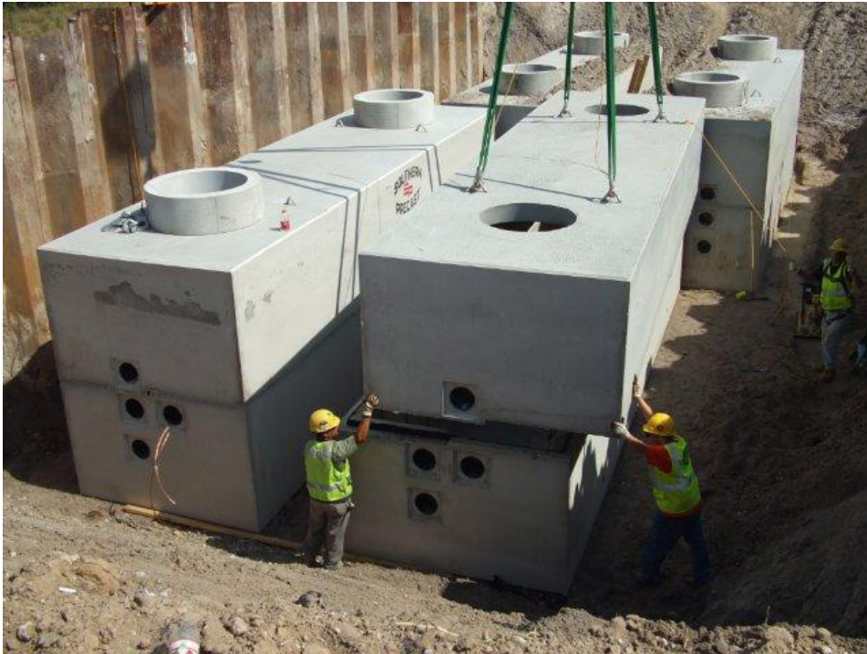
Splicing vault installation (Source: POWER Engineers)
