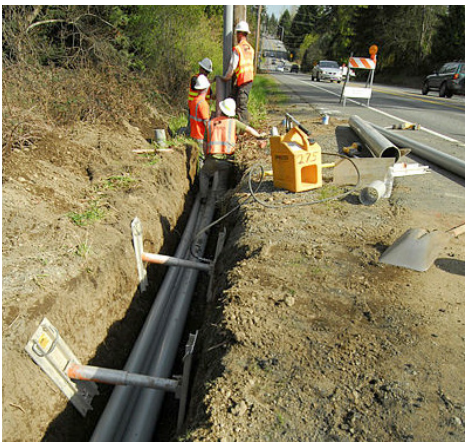
Underground distribution cable replacement
